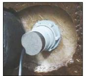
The new design of In Pool temperature sensor installs in the same manner as the existing products. Fit the body (number 1 in the diagram) into the hole in the shell and secure with the lockring (2). Use silicone or similar for a water proof seal. Slide in the sensor slug (3) into the body, there should be enough
