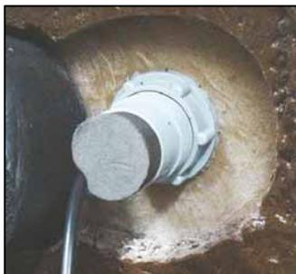
The new design of In Pool temperature sensor installs in the same manner as the existing products. Fit the body (number 1 in the diagram) into the hole in the shell and secure with the locking ring (2). Use silicone or similar for a water proof seal. Slide in the sensor slug (3) into the body, there should be enough silicone grease to make it water tight. It is important that the foam plug is pushed as far as it will go into the body.
